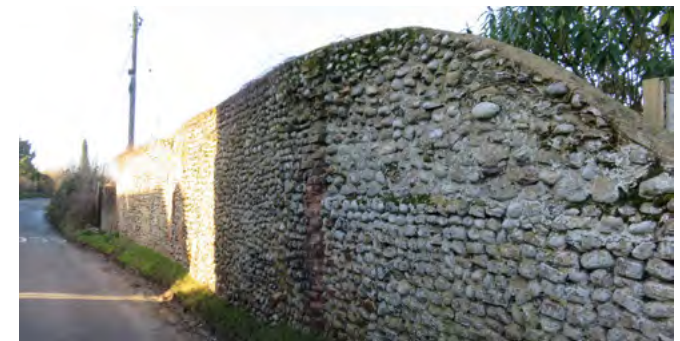
Flint walling associated with Green Farm, Blakeney Road
