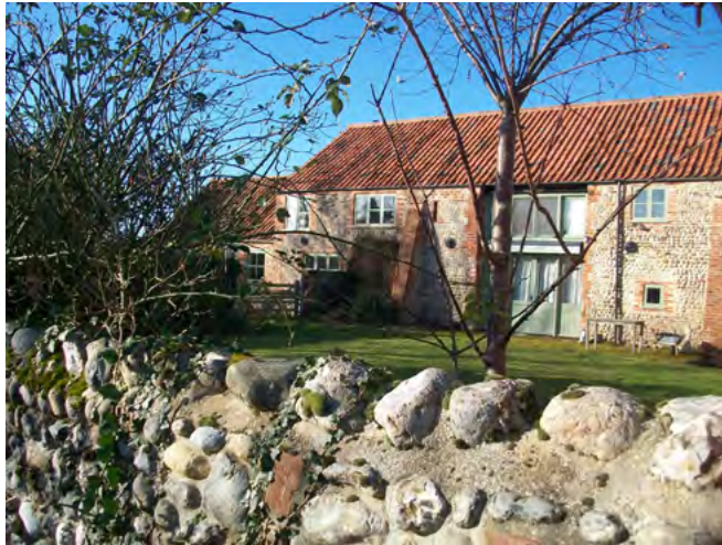
The converted Church Farm Barn, Chapel Lane
