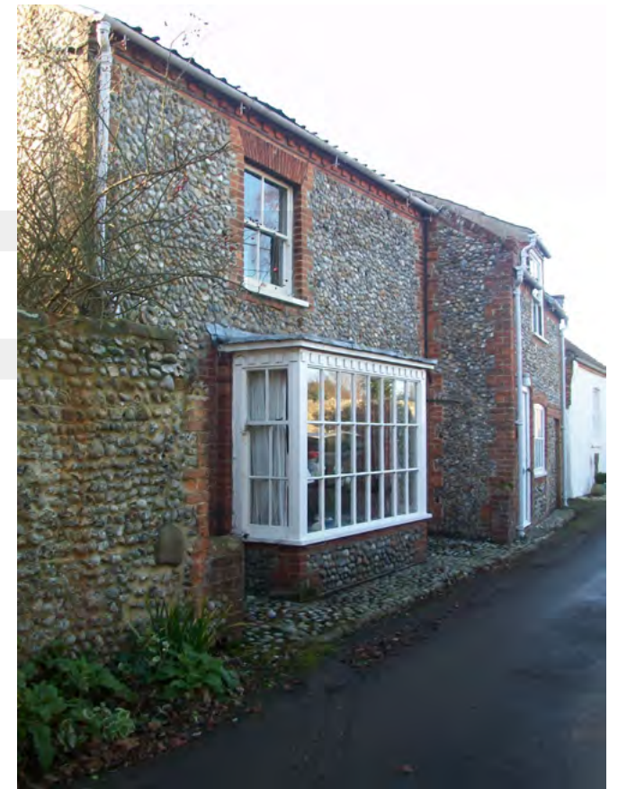
Possible historic shop front on Chapel Lane
