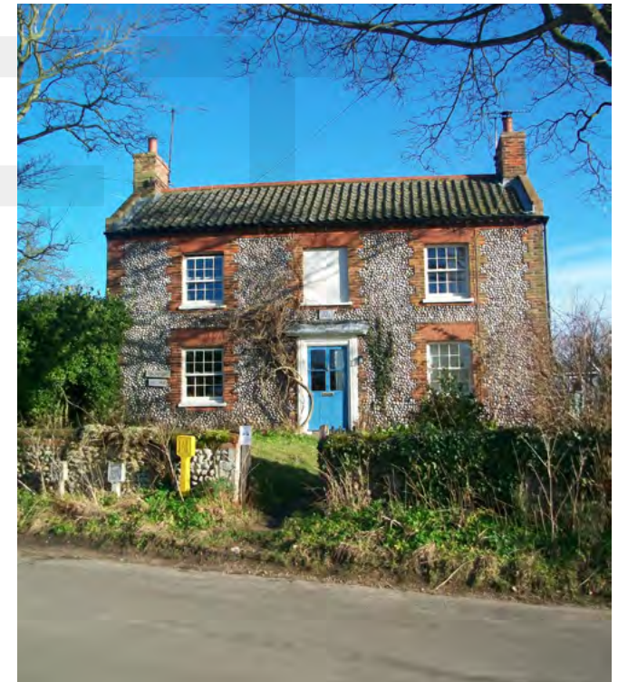
Detached historic brick and flint house, Sycamore House, The Street
