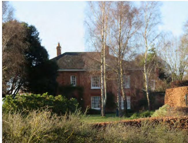
Eighteenth century brick built detached house, the Old Rectory, Bridgefoot Lane
