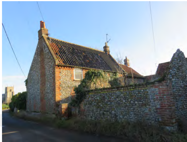
Green Farmhouse and shed, Blakeney Road
