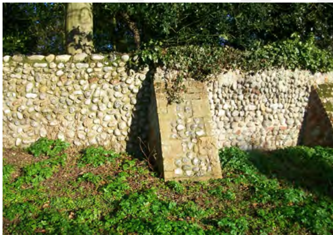
Flint walling with brick and flint buttress, Hall Lane
